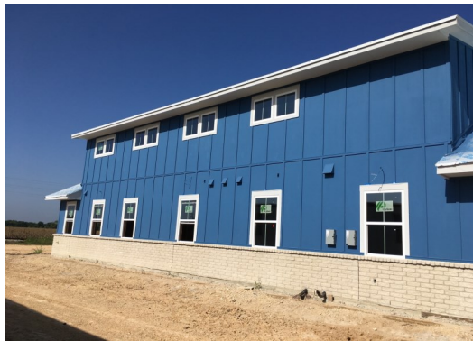
July 18, 2018— Back of building
